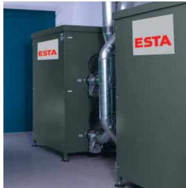
Two side channel blowers as part of a central dust extraction system
