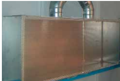
Extraction wall with perforated metal insert
