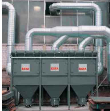
Modular filtration unit
