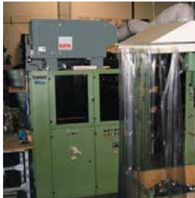
Oil Mist Separator in operation
