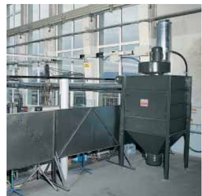
Modular extractor DUSTEX in a metalworking application
